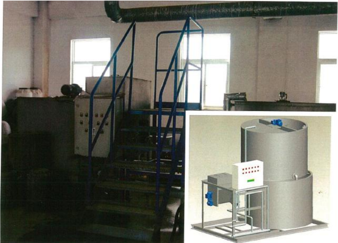
PTB type polymer dosing system
