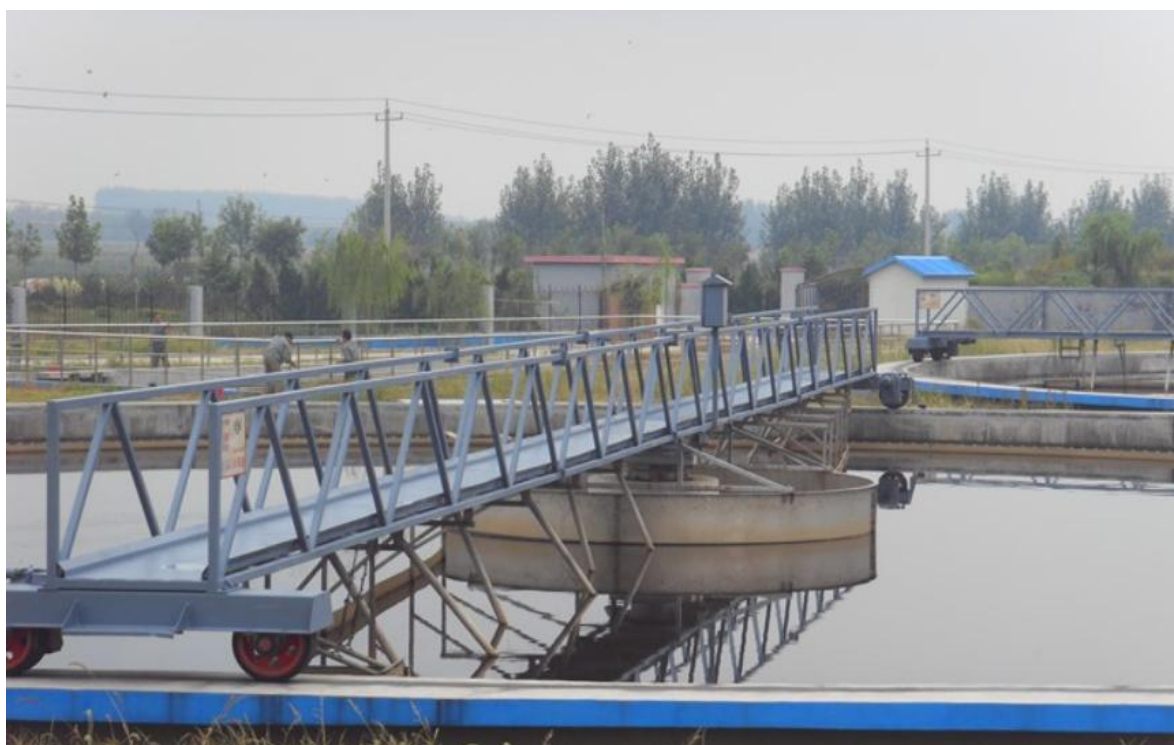
QG type Traveling Bridge Scraper
