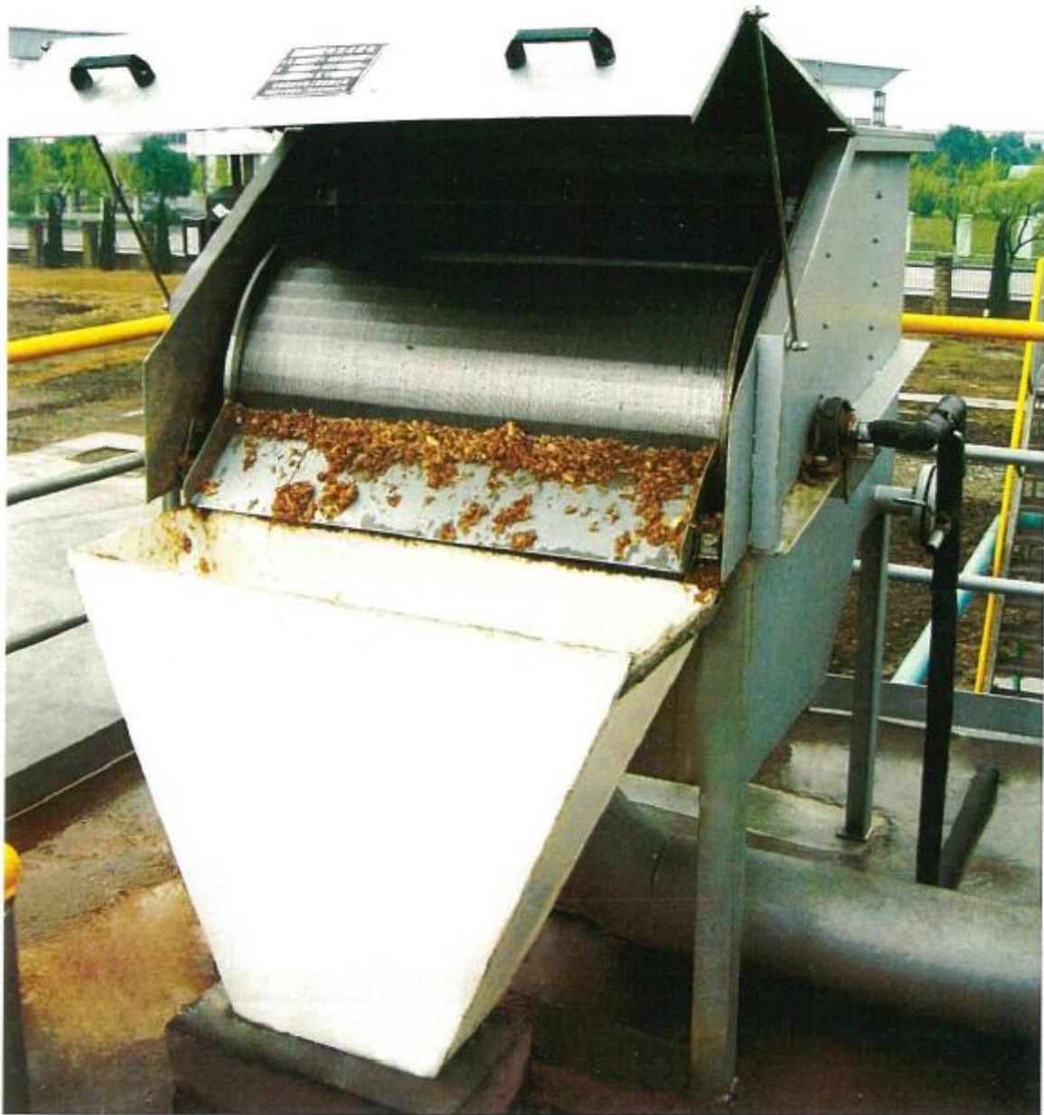
RSM Type Rotating Drum Screen
